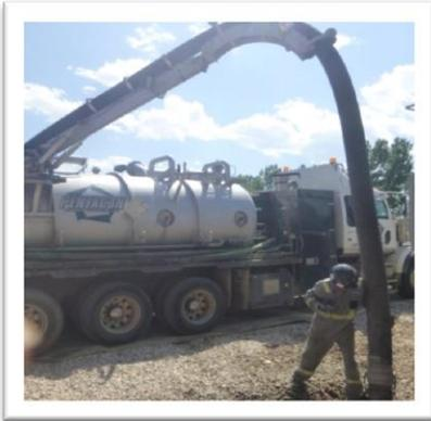
The top layer of surface/fire quenching stone was removed by Hydrovac truck (left). Some areas were dug by hand (right).
