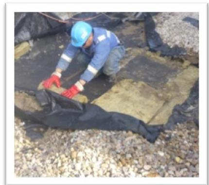
Woven geotextiles and sand were removed. The Absorbent layer was rolled up and placed in plastic bags for disposal (right).
