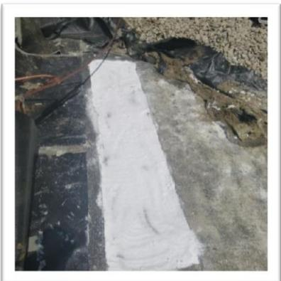
Some Albasorb was spread on the sand layer, a strip of oilmat was placed overlapping the existing oilmat, and more Albasorb was spread on top and around the seams of the new oilmat strip.
