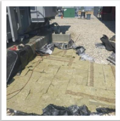
New layers of non-woven, adsorbent, woven, and sand were installed only over the affected areas where material was removed (left & right). The containment was then re-filled with fire quenching stone and cover stone. (below)
