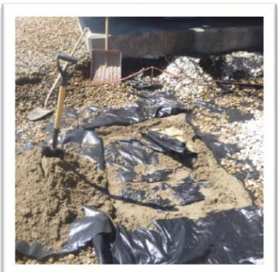
An inspection test area was established in the area that the spill occurred. The top and bottom layers of woven geotextile, the 50mm of sand, and some of the absorbent layer were found to be saturated in this area (left).
